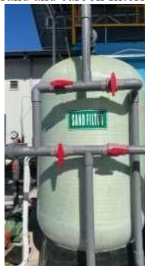
Figure 10. Sand and carbon filters
